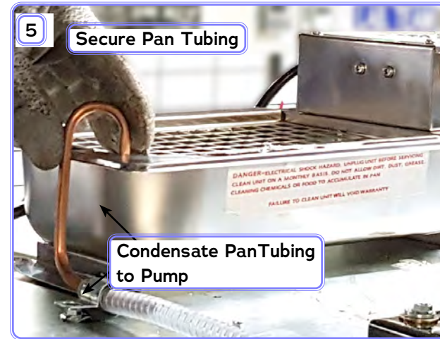
Condensate Pan (Installed on Top of Case)
