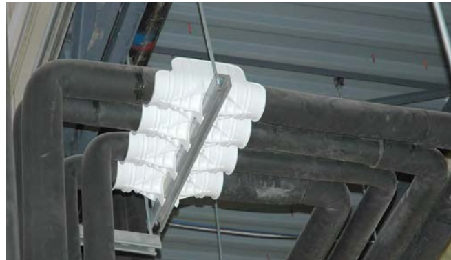
Ceiling Run with Supports
