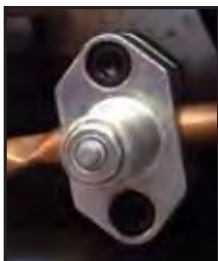
refrigeration line tapping valve
