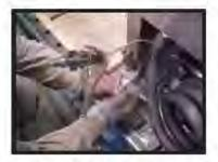
Once it is ensured that the service port does not leak, braze it closed. Remove all service ports. If a Schrader valve was used on the compressor service tube, it must be removed and the previous steps followed to braze the service tube shut.
