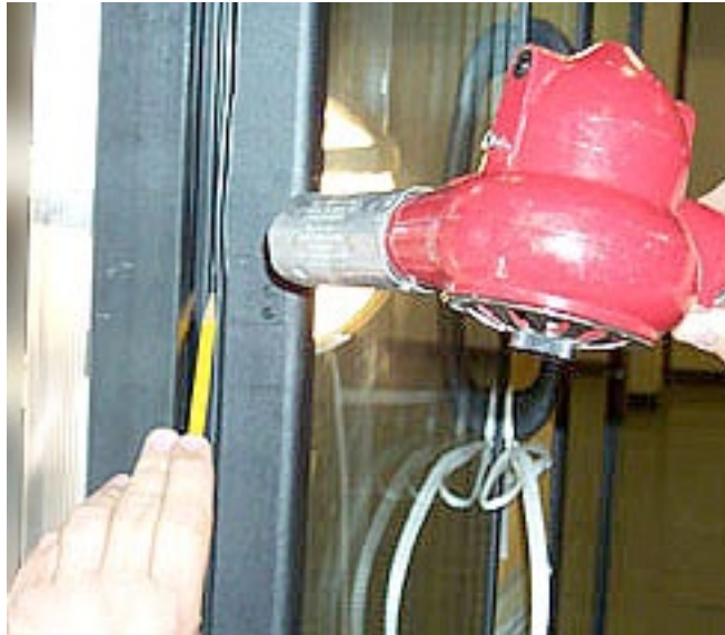
Pulling Gasket Into Place With a Pencil
