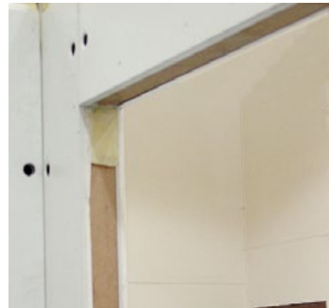
Standard Reinforced Opening
