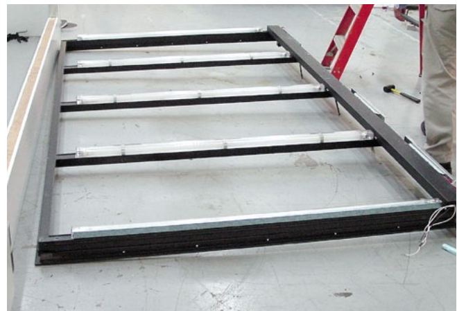
Unpack Frame and Lay Face Down
