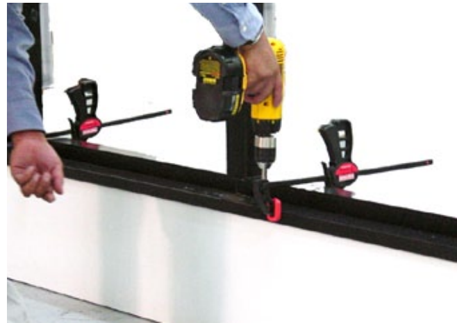
Fasten the Frame Bottom
