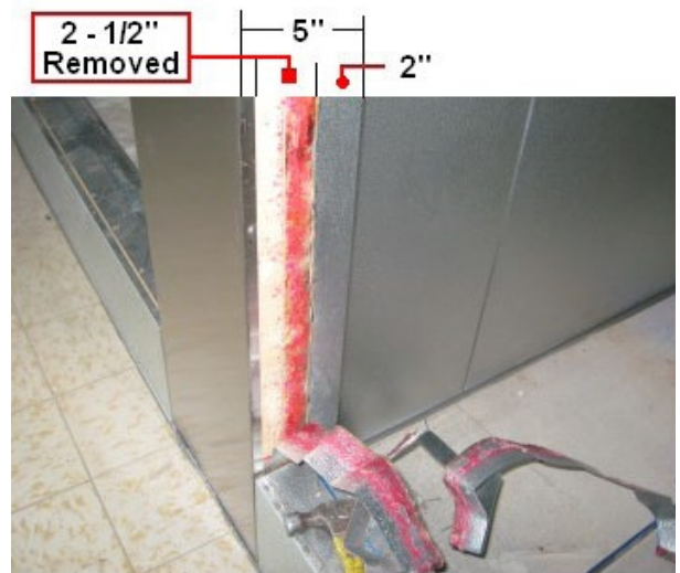
Removal of Metal around Opening
