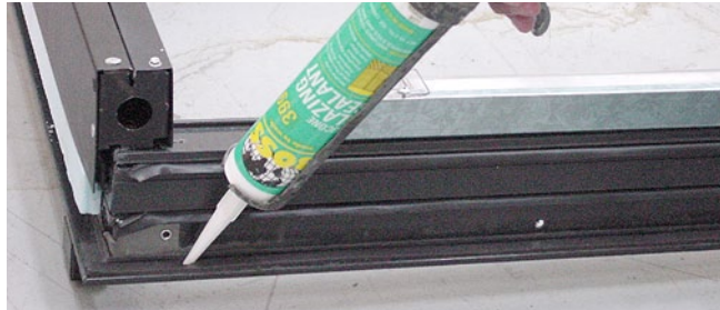
Apply Silicone Sealant
