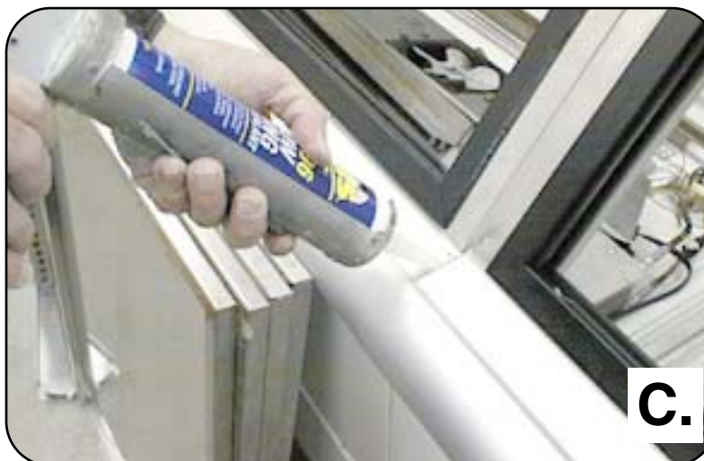
Figure 15. Sealing Case Joints
