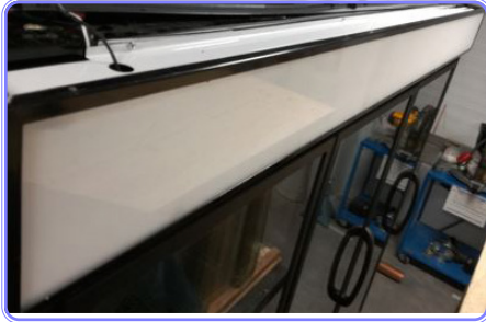
Display Slides out to access Wireway
