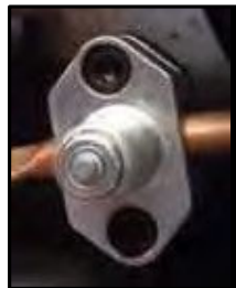
refrigeration line tapping valve
