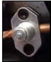
refrigeration line tapping valve
