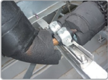
The suction line and liquid line need to be insulated to the evaporator. Install clamps to mitigate vibration.
