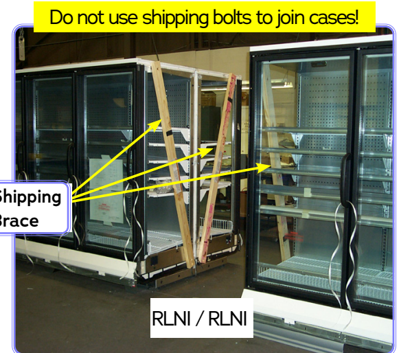
Remove Shipping Braces
