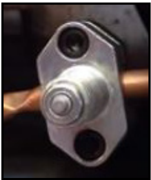
refrigeration line tapping valve
