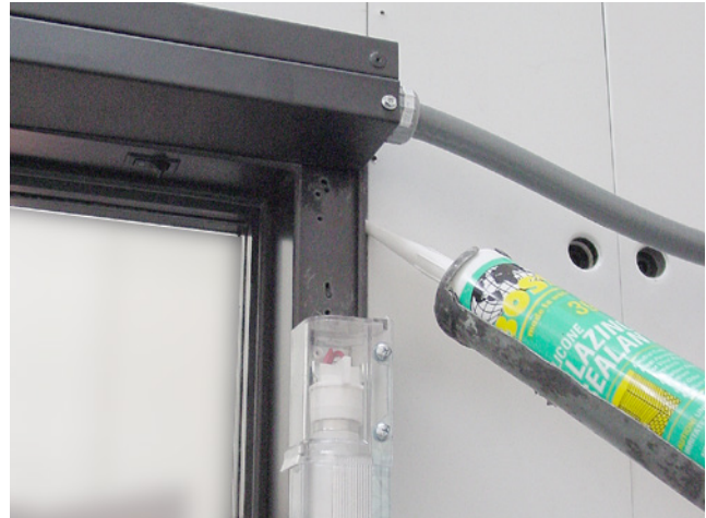
Apply Silicone Around Frame
