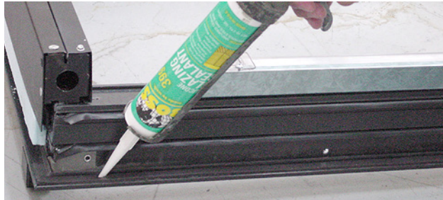
Apply Silicone Sealant
