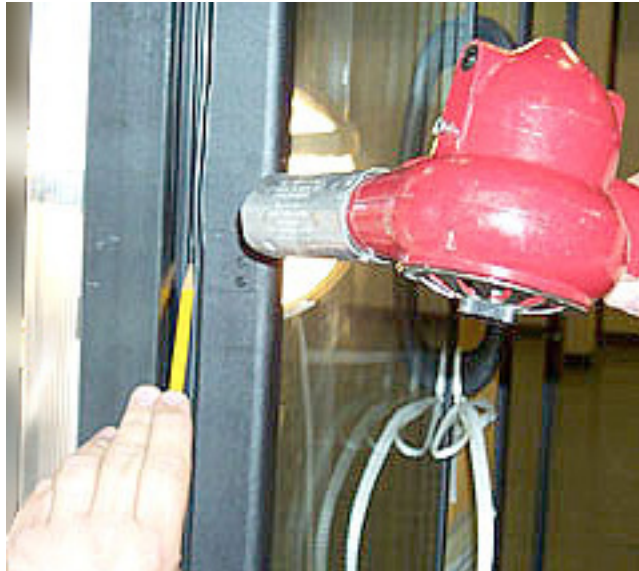
Pulling Gasket Into Place With a Pencil
